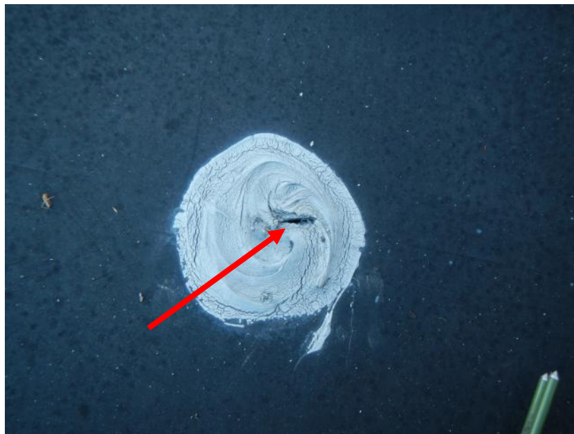
Observation Photograph 4 – View of EPDM membrane opening with surface applied sealant.
