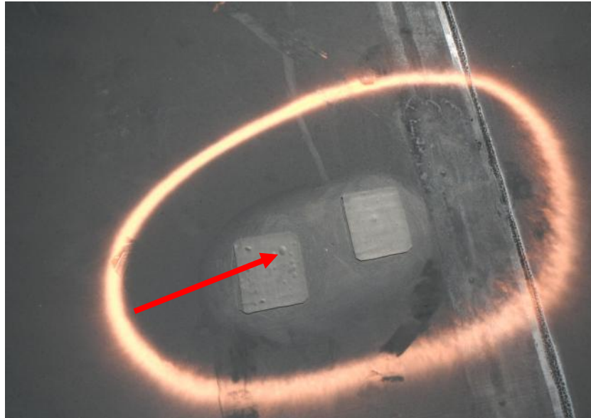
Observation Photograph 5 – View of typical patches on S2. Arrow indicates blisters in patch.
