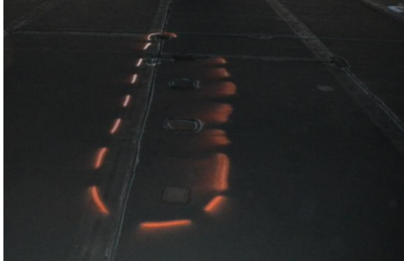
Observation Photograph 3 – View of typical patching throughout the roof system and paint marking for further assessment.
